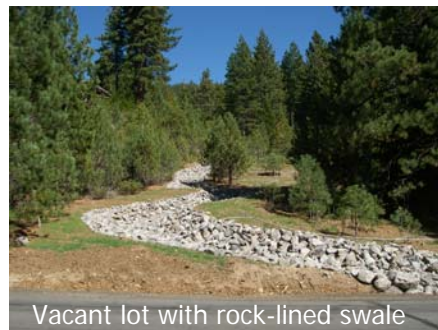
Infiltration swale along road
